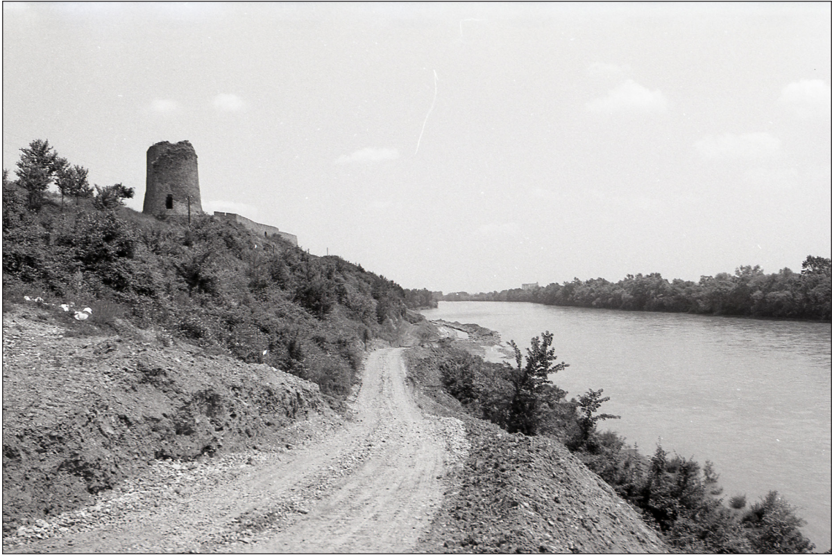
Figure 1. Dobor during construction works in 1978 (photo: B. Belić).
